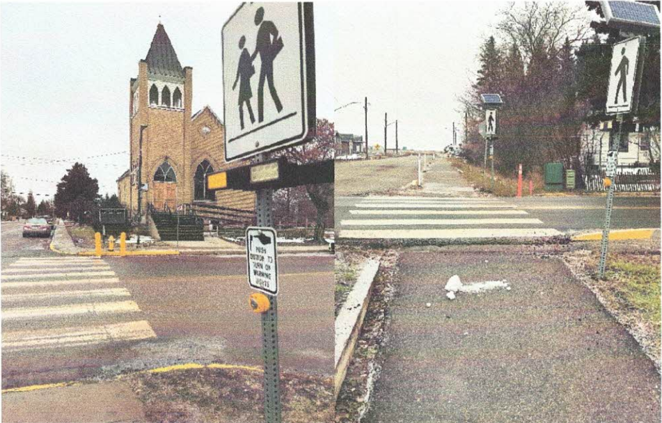
Addition of 3 sets of lighted crosswalks for the community.
